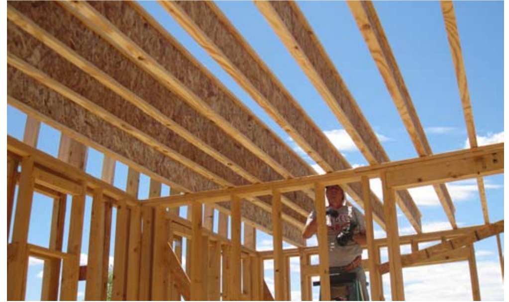
Lightweight I-Joists installed in place of traditional solid timber joists
