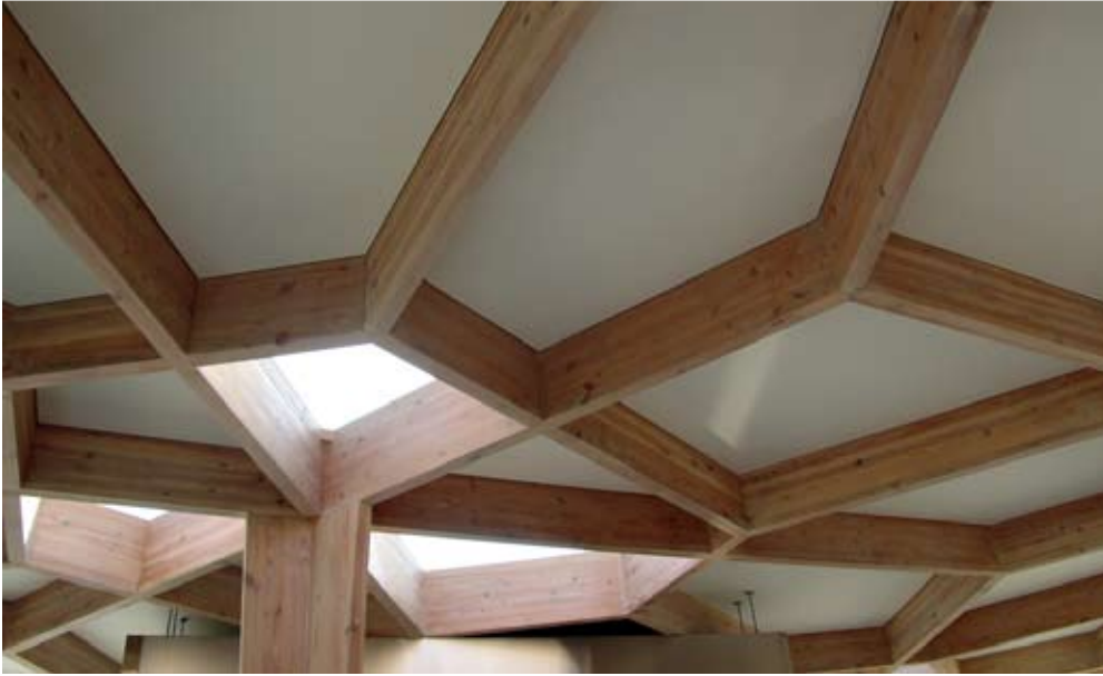
Glulam beams in use in the Sumika Pavilion by architect Toyo Ito
