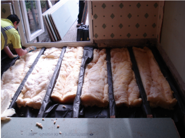
150mm of mineral wool insulation fitted between floor joists
