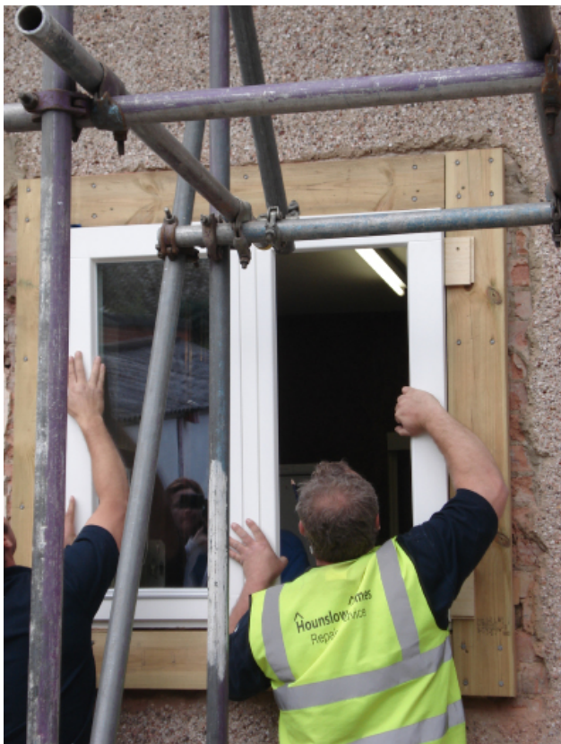
Installing triple glazed passivhaus windows with timber surround
