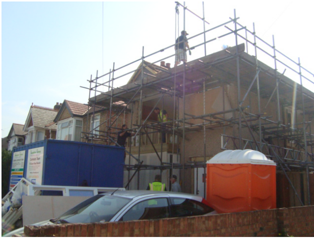
Timber frame construction of bay window area
