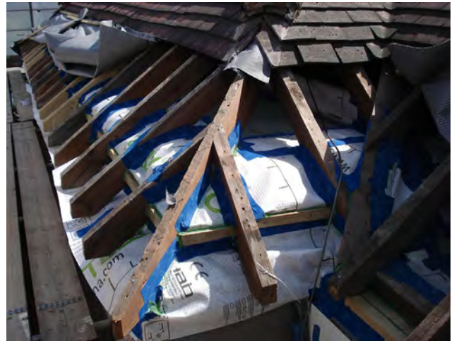
Continuous airtight layer between parge coat to walls and airtight layer in attic
