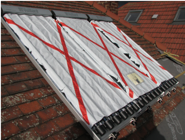
Solar thermal array installed
