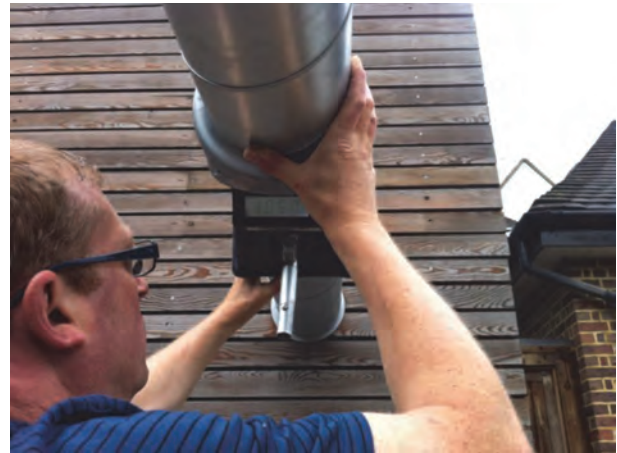
Figure 7: Ventilation system testing
