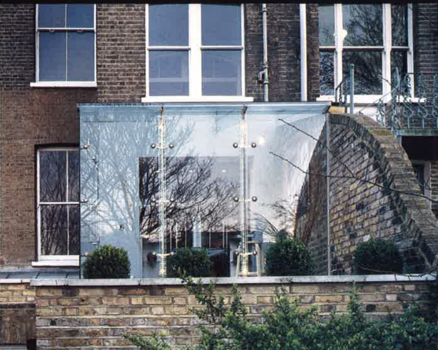
Fig. 8.2 Conservatory at a house in Clapham, South London (courtesy Bere Associates/Michael Heyward)
