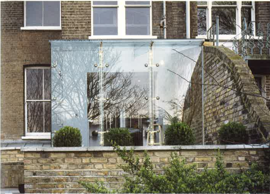
Fig. 4.13 Conservatory at a house in Clapham, South London (courtesy Bere Associates/Michael Heyward)
