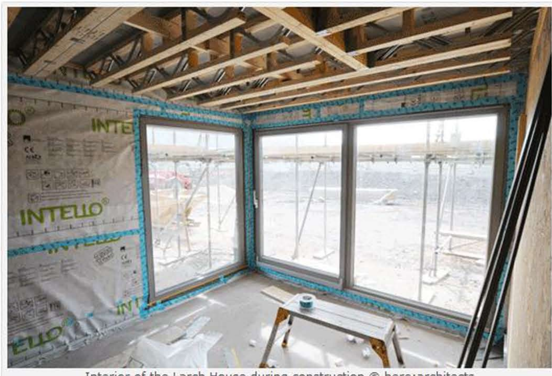
Interior of the Larch House during construction © bere:architects
