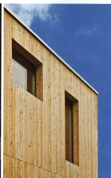
Far left: Airtightness tape being applied to window frames before site installation (the opening light has been taken out to make handling during installation more manageable). Image courtesy of Bere architects
