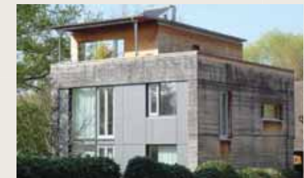
Passivhaus standard housing exemplar (above) in Freiburg, Germany, using Bayer's super-airtight window.
