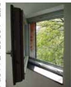
The windows open inward to avoid being exposed to rain.
