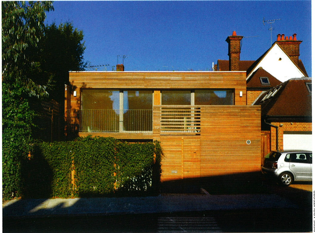
Above Structured panels with cladding were prefabricated
